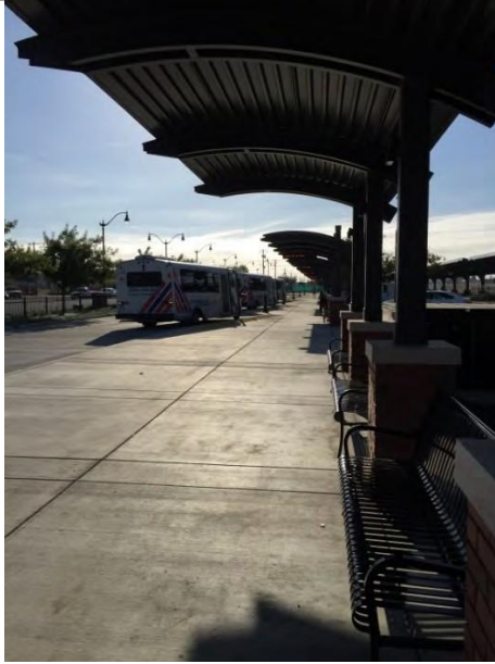
Manteca Transit Center bus bays
