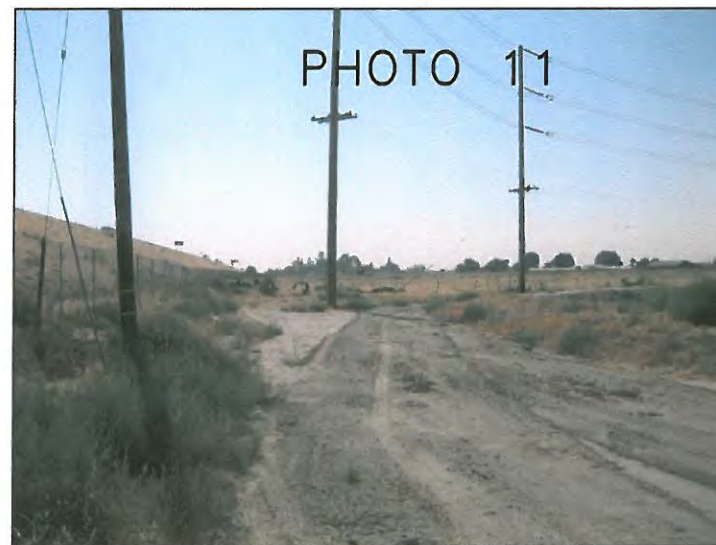
SERVICE ROAD FACING EAST TO MCKINLEY AVENUE OVERHEAD UTILITIES NORTH OF SERVICE ROAD
