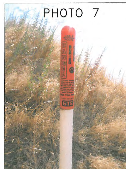
MCKINLEY AVENUE—FACING EAST BURIED UTILITY CABLE SIGN FOR GTE
