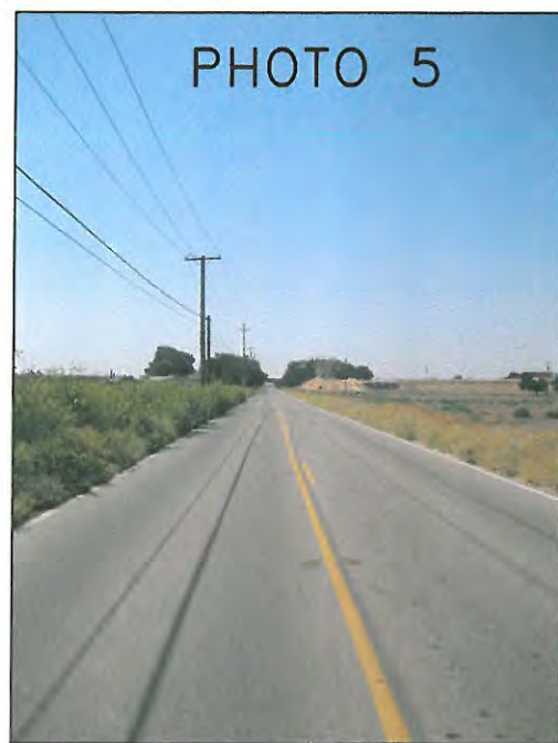
MCKINLEY AVENUE—FACING SOUTH OVERHEAD UTILITIES ON EAST SIDE OF ROAD
