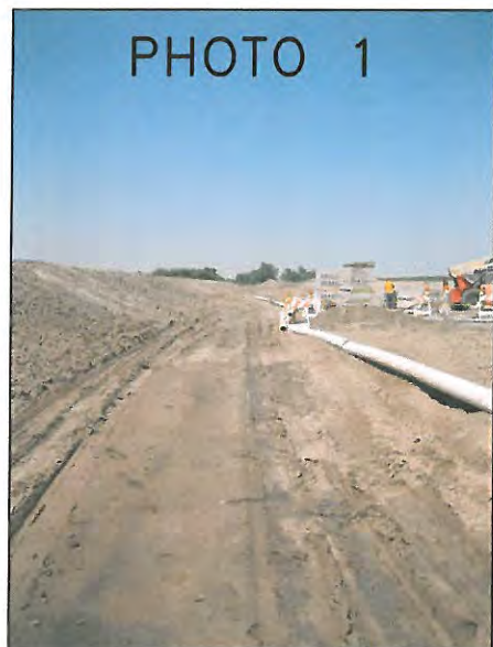
WQCF—FACING WEST BETWEEN SECONDARY EFFLUENT STORAGE POND AND CHEMICAL BUILDING
