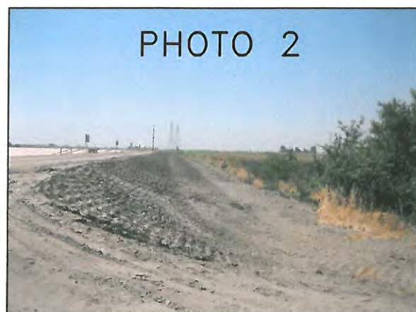
WQCF—FACING SOUTH WESTERN LEVEE OF ECKERT POND
