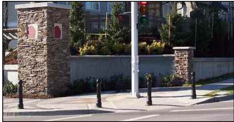
Use of bollards to separate pedestrian area from the street
