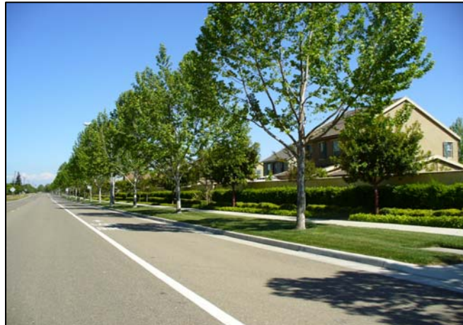
Decorative masonry enhances this soundwall
