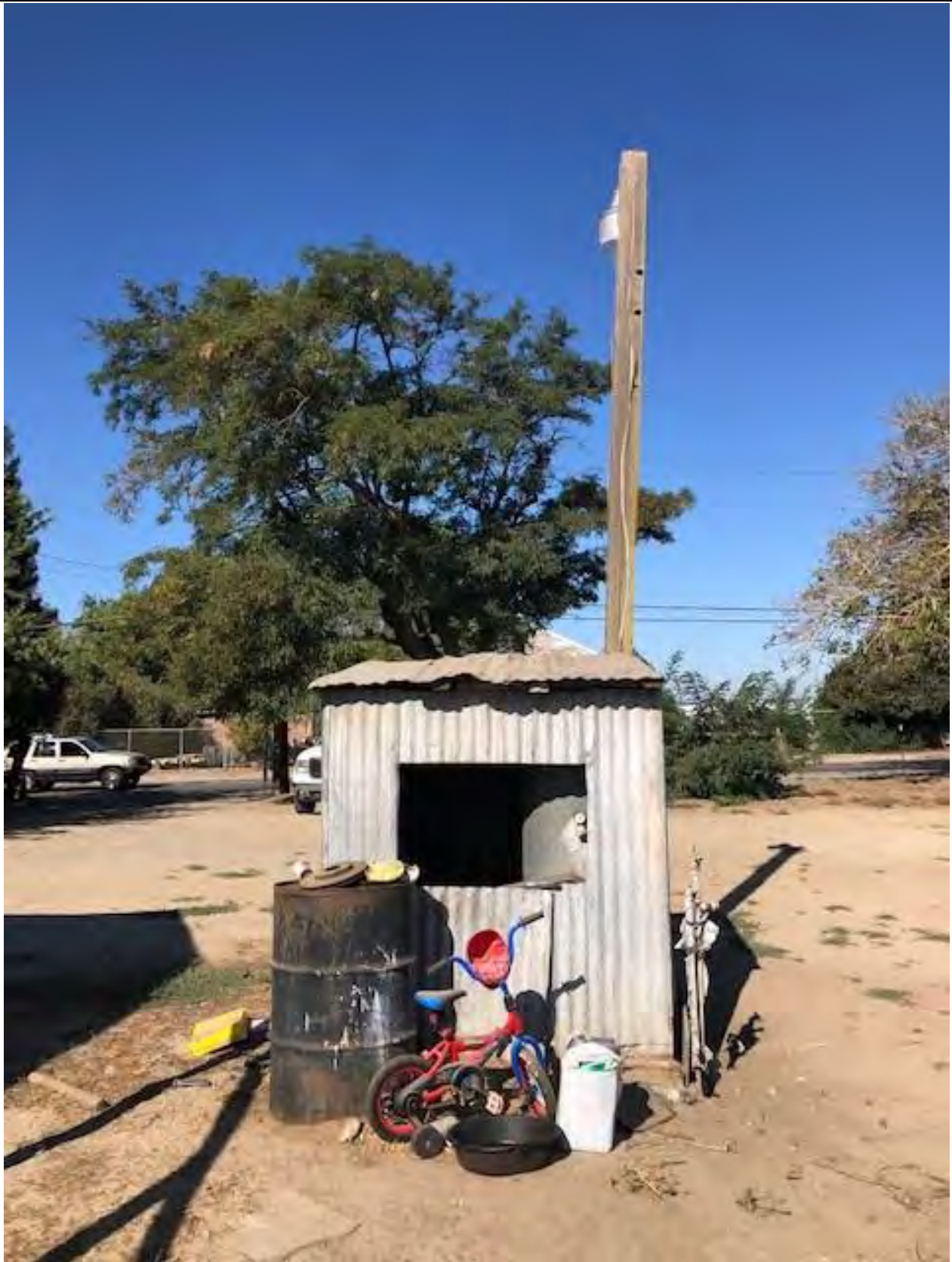
K) View looking west of the east facing façade of Building No. 2. 8/31/2021. Acc. #21-3599.
