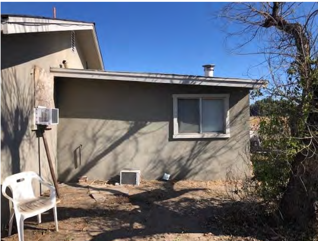
D) View looking north of the partial east facing façade of the residence (left), south facing façade of the addition (center). 8/31/2021. Acc. # 21-3592.
