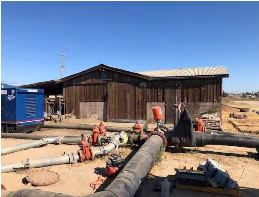
H) View looking north of the south facing façade of Building No. 1. 8/31/2021. Acc. # 21-3602.
