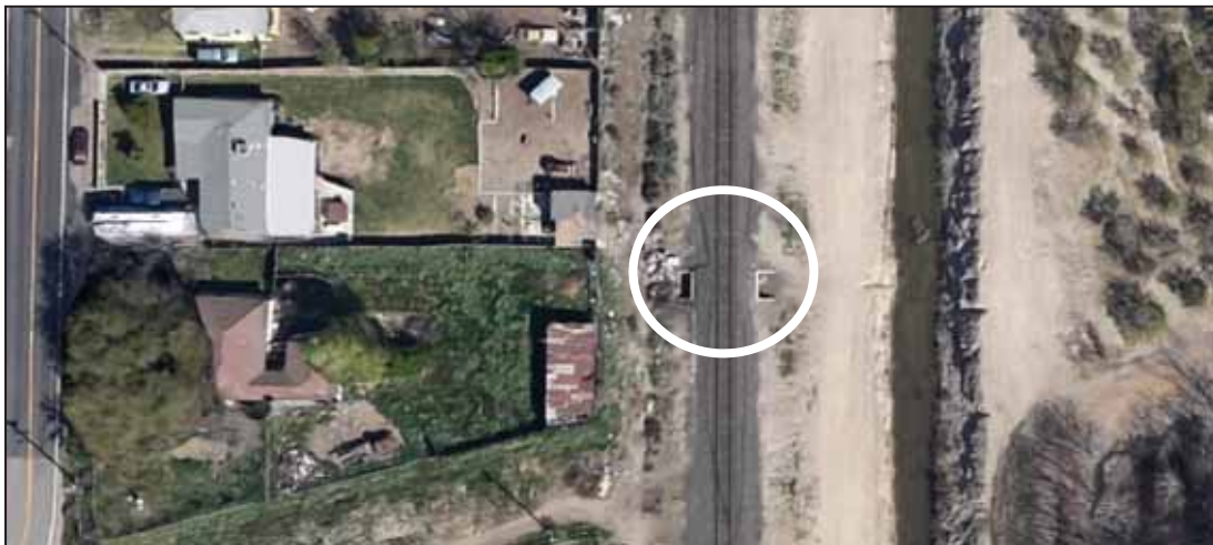
Figure 21. Aerial photo of the added culvert near S. Janet Rd.
