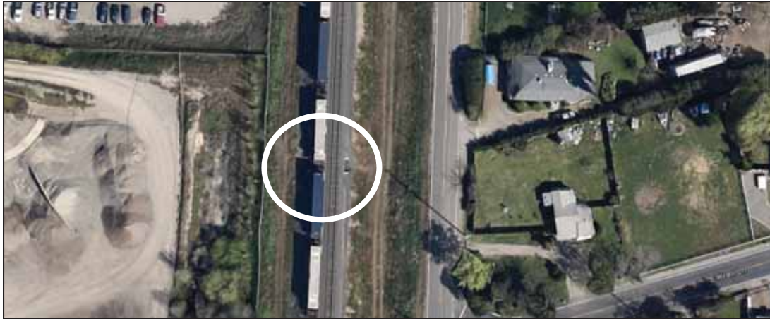
Figure 22. Aerial photo of the added culvert near E. Krell Lane
