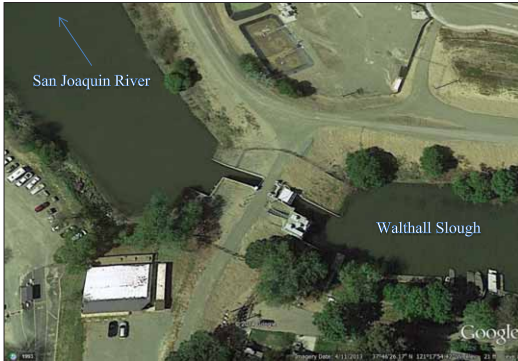
Figure 3. Walthall Slough gate control structure.
