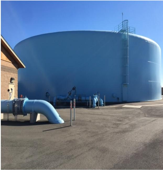
Atherton Drive Storage Tank and Booster Pump Station. Five variable frequency pumps, onsite treatment, and a 3.7 million gallon tank serve peak water demands. The facility was completed in 2014.
