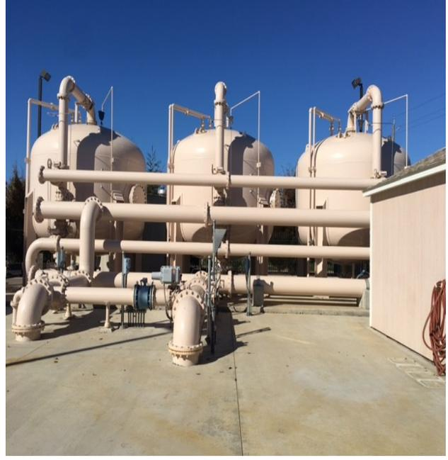
Wells 13, 19, and 21 have local treatment facilities for arsenic removal, but nitrate, manganese, and TCP 123 are treated at a central treatment facility, shown above, where blending with surface water is performed.
