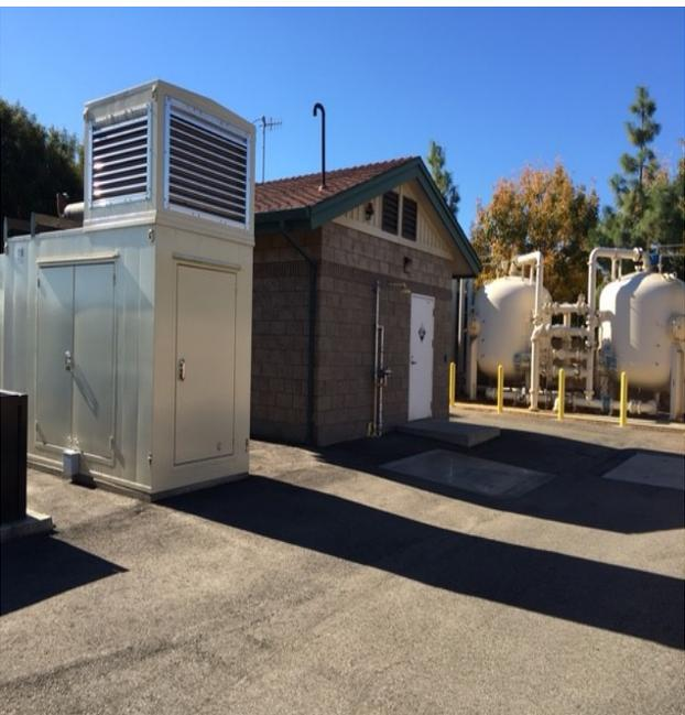
Well 24, off of Van Ryn Avenue, is one of several City wells with onsite manganese green sand filtration to remove arsenic, which is a problem at deeper levels of the aquifer.
