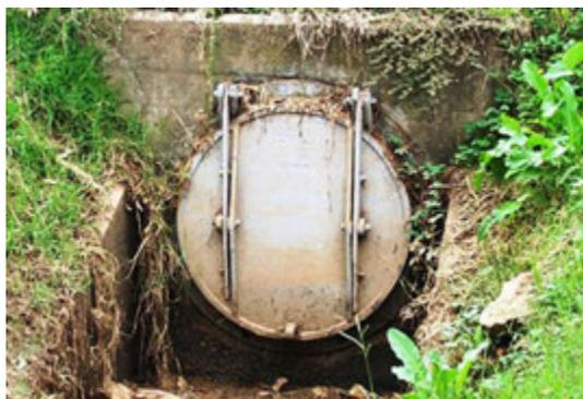
**Figure 2.65** UNACCEPTABLE vegetation around flap gates in earthen levee. (OK)
