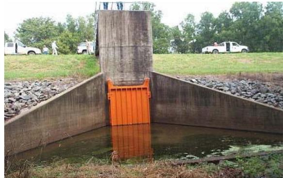
**Figure 2.63** ACCEPTABLE culvert gate. (LA)
