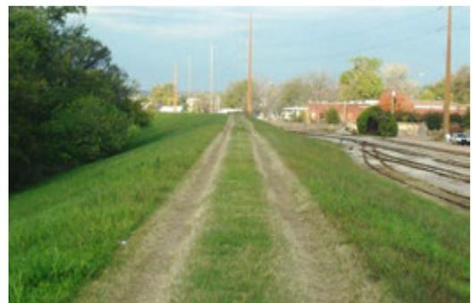
**Figure 2.39** *UNACCEPTABLE* rutting in levee. (OK)
