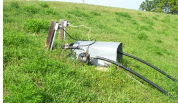
**Figure 2.8** UNACCEPTABLE encroachment. Piping for lawn irrigation system drilled through levee without approval. (ND)
