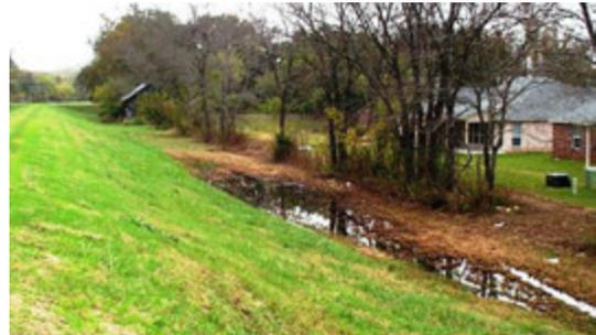
**Figure 2.53 UNACCEPTABLE interior drainage** *at the toe of an earthen levee. (OK)*
