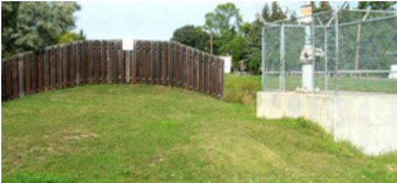
**Figure 2.11** UNACCEPTABLE encroachment. Residential and rural fences crossing the levee. (ND)
