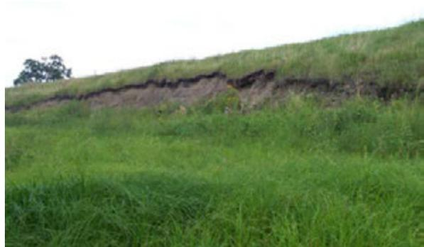
**Figure 2.17 UNACCEPTABLE** earthen embankment failure. (MN)
