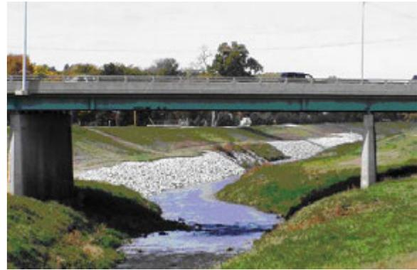
**Figure 2.26** ACCEPTABLE riprap for erosion control. (NE)
