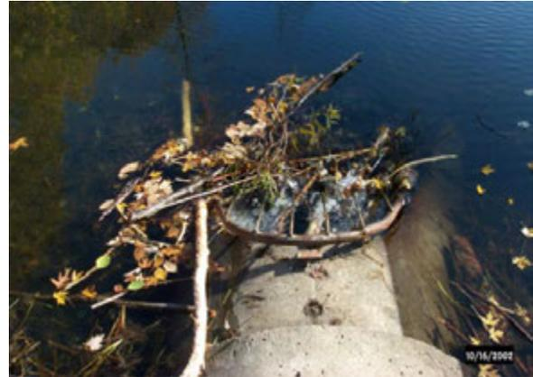
**Figure 2.22** Beavers attempting to block the culvert passing through a gated embankment. (MN)
