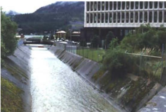
**Figure 2.74** ACCEPTABLE concrete lined channel. (AK)
