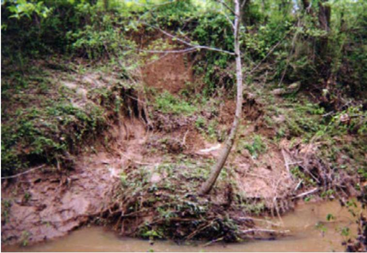
A related slope failure/ stability problem involves trees growing on or near the channel or levee slopes. It's very important to prevent tree growth near levee or channel embankments, because when the roots of these trees decay they leave voids in the soil, which allow water to quickly saturate the slope and cause a slope failure. Trees can also be uprooted and deflect flood flows into the embankment, accelerating the erosion of the bank.
