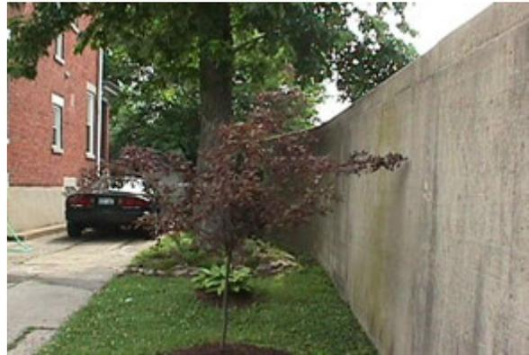
**Figure 2.52 UNACCEPTABLE.** *Trees growing too close to floodwall. (KY)*
