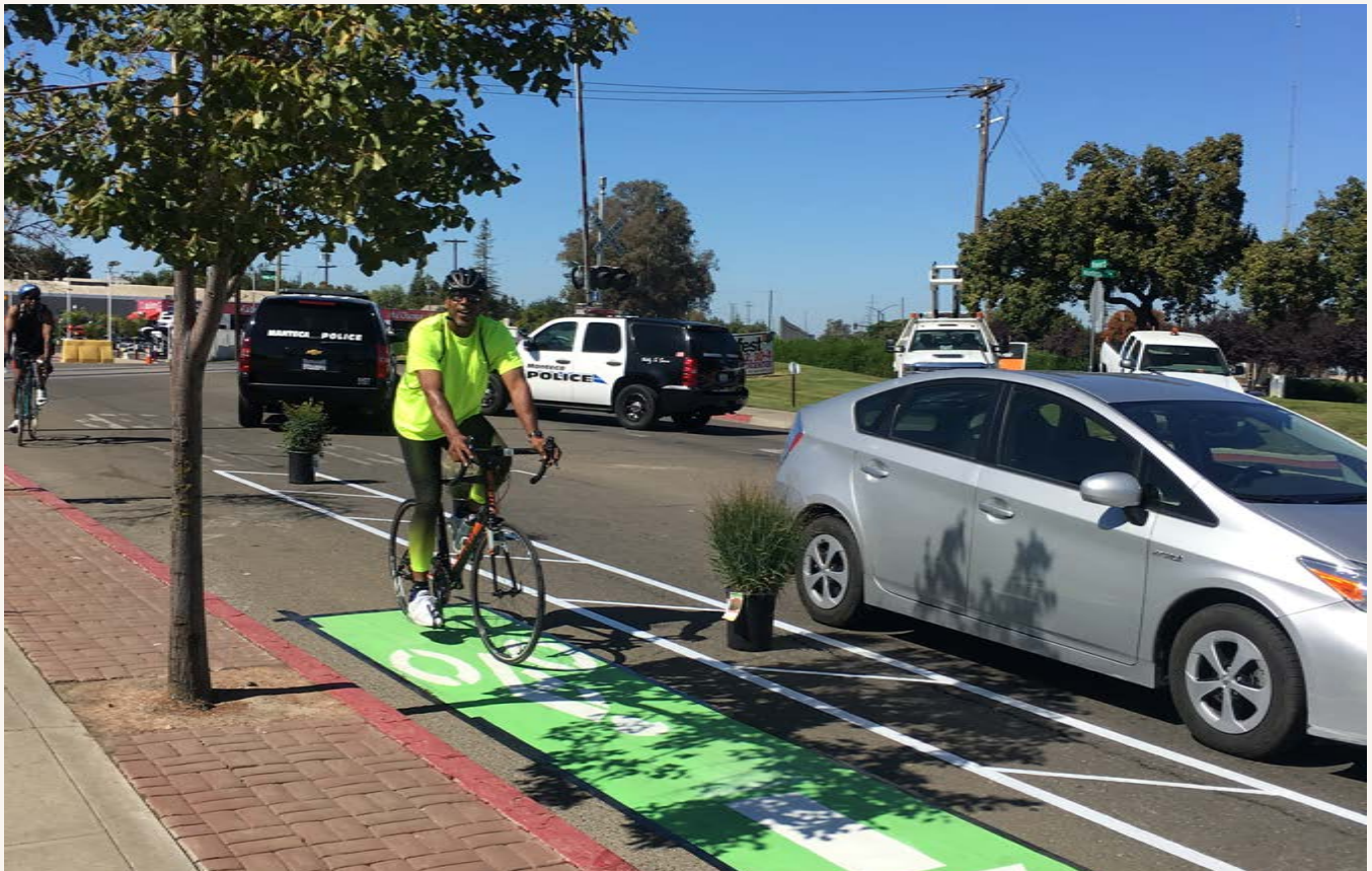
Temporary parking protected bike lane on Yosemite Avenue
