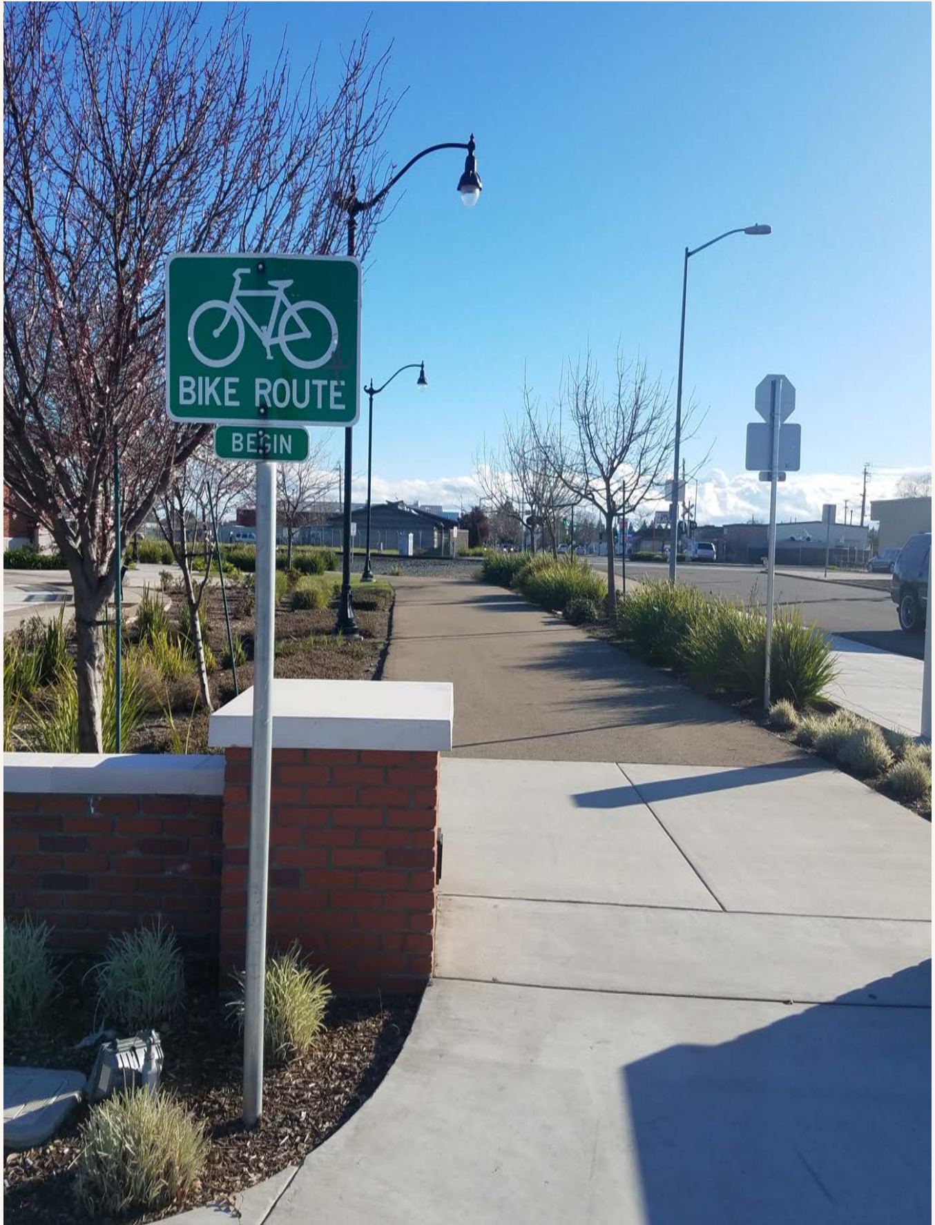
Bike Route at the Manteca Transit Center
