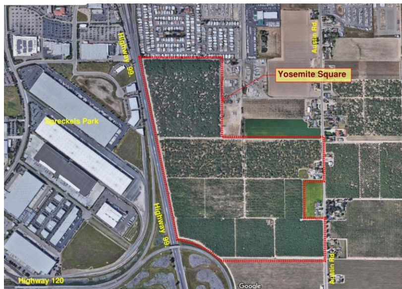
Project aerial – Existing conditions
