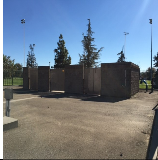
The sewer lift station at Woodward Park, along Buena Vista Drive, will be replaced in the near future when a new gravity line servicing the area is installed.
